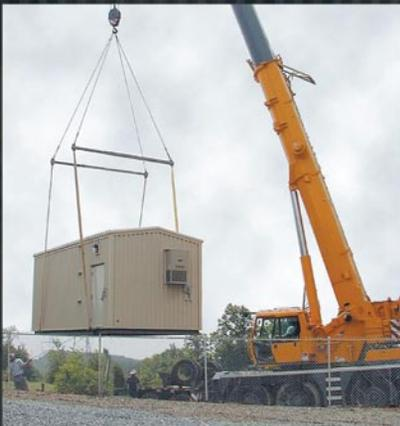
**Preassembled Collector and Interconnect Substation Control Buildings**
