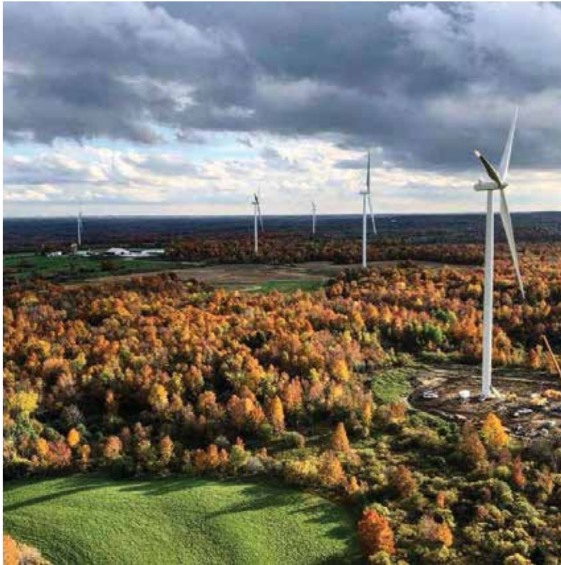
The Copenhagen Wind project is the first wind project that RES has self-performed in the State of New York and consists of 40 Vestas V110 2.0 MW turbines. (Courtesy: RES)
