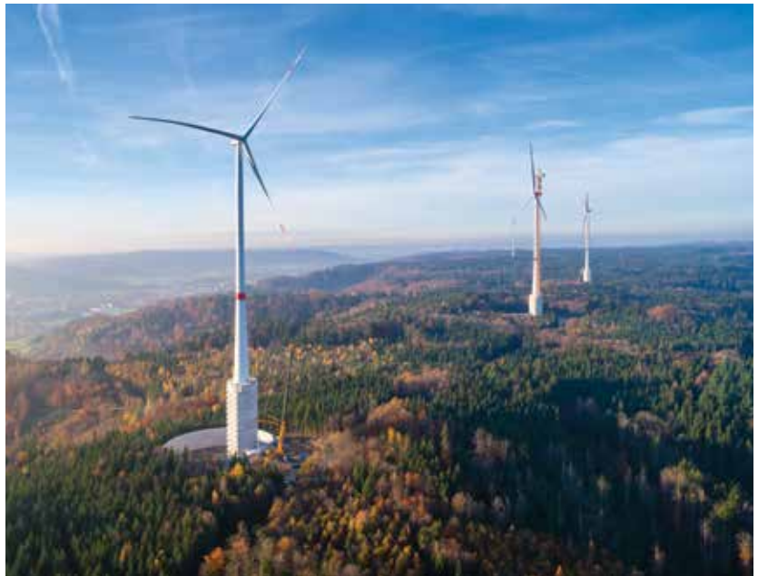
Max Bögl built the world’s highest onshore turbine in Gaildorf, Germany, with a 178-meter hub height. The turbines are part of Max Bögl’s Water Battery storage project. (Courtesy: Max Bögl Wind AG)
