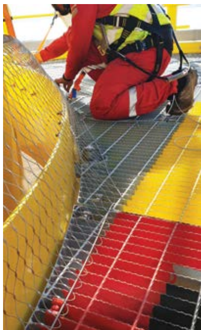
The Dropsafe Net is a stainless-steel mesh net engineered to securely enclose and tether overhead fixtures, mitigating the risk of them falling and threatening the safety of personnel. (Courtesy: Dropsafe)
