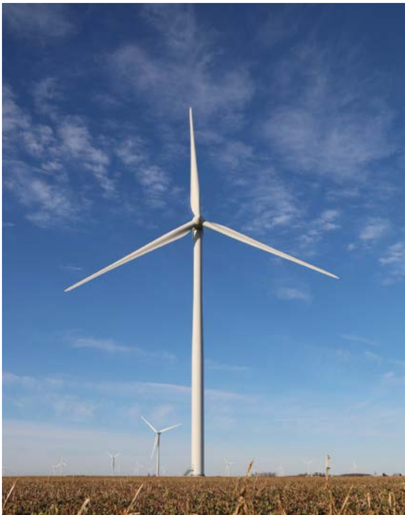
Siemens Gamesa will repower the Iowa project with 163 SG 2.7-129 and 18 previously sold SWT-2.3-108 wind turbines. (Courtesy: Siemens Gamesa)
