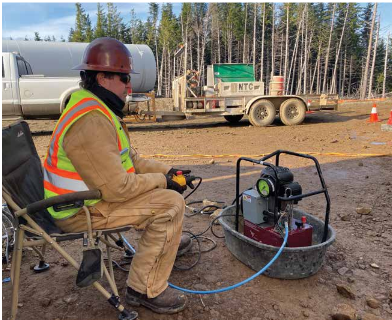
Associate Drew Yancey operates the tensioning pump. (Courtesy: NTC Wind Energy)
