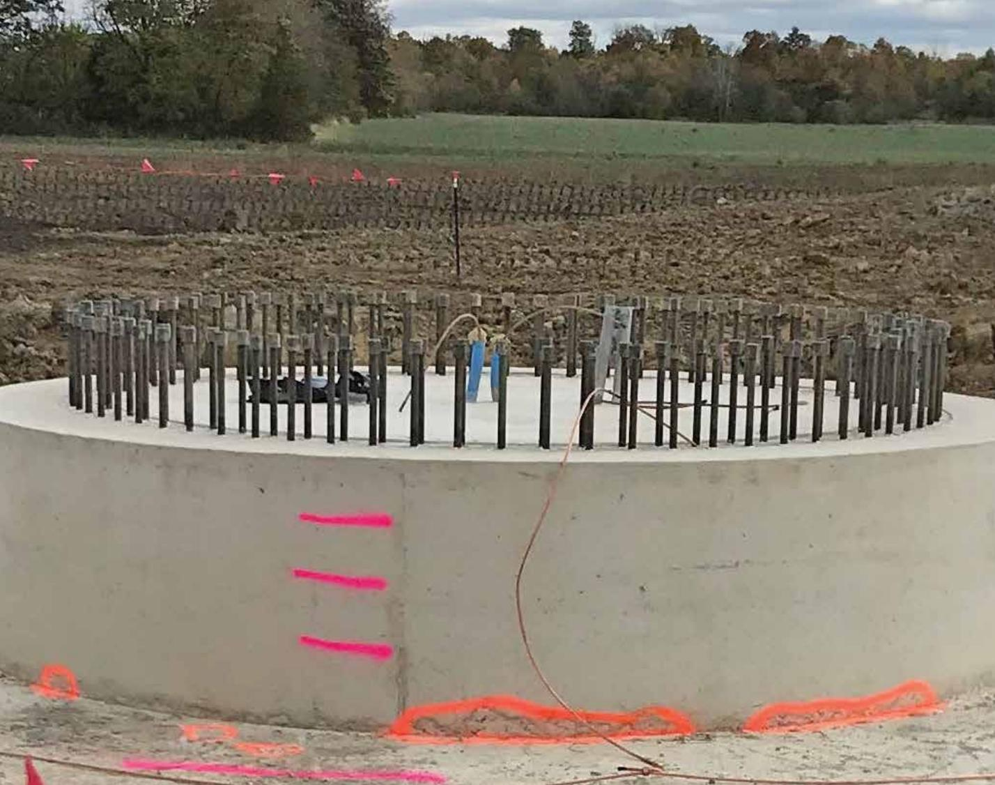
A recently completed foundation where Dyson's anchor bolts were used. (Courtesy: Dyson Corporation)
