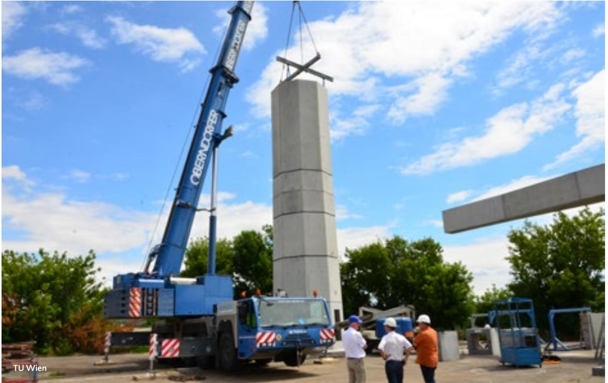
A team led by Professor Johann Kollegger at the Institute of Structural Engineering at Technische Universität (TU) Wien has developed a new tower construction method wherein double-wall elements are joined together on the ground to form large double-walled concrete rings. These rings are then lifted up with a crane, stacked one on top of the other, and filled with concrete. This technique results in a construction method for wind tur-
