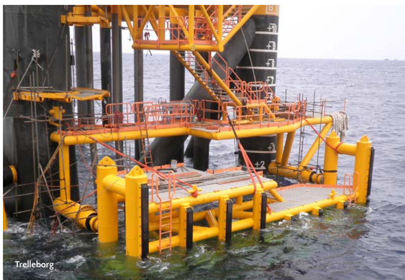
Trelleborg’s boat landing system on site.
