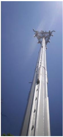
Fig. 2: A reinforced monopole with blind bolted, Pole Max structural channel.
