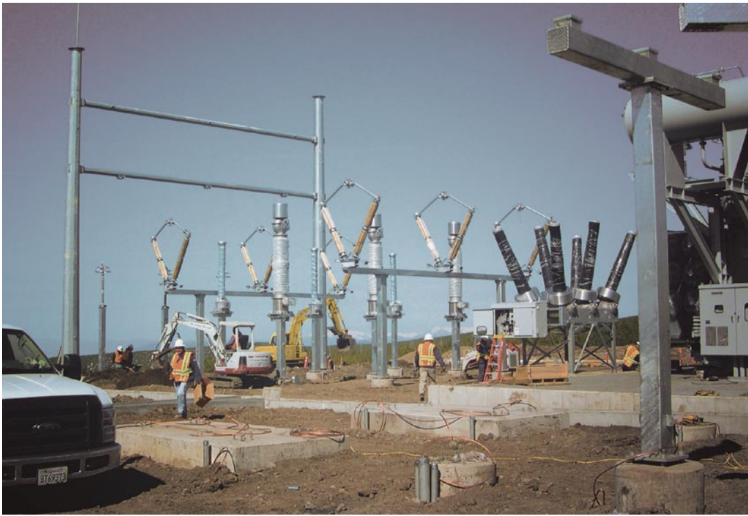
Fig. 2: The Hatched Ridge Wind Farm, under construction.
