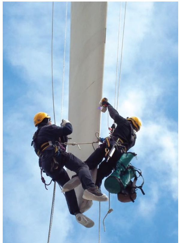
Fig. 4: Repair using handheld UV lamp.
