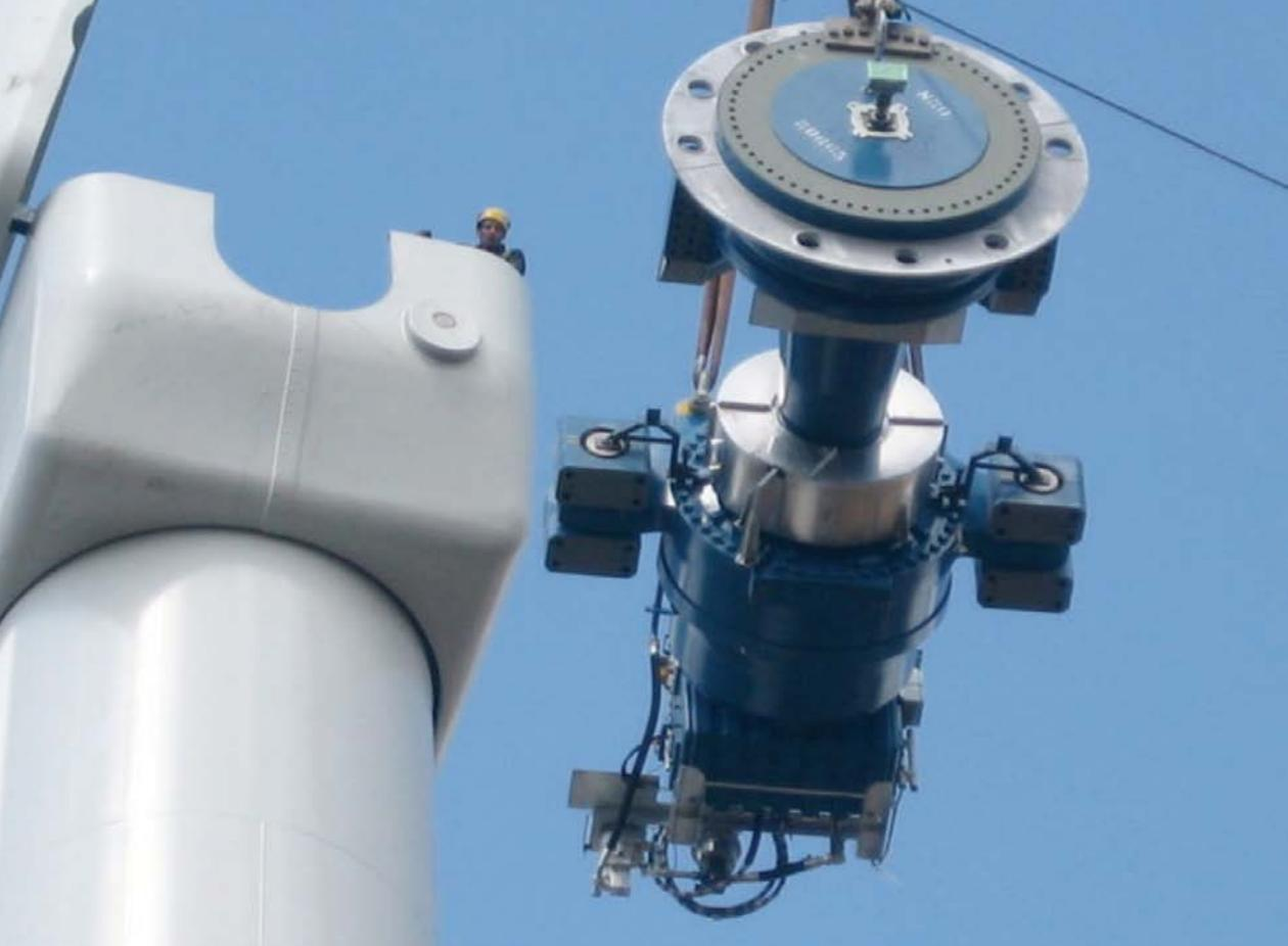
**Fig. 1: Gearbox, rotor shaft, and disk brake assembly (Scout Moor Wind Farm Construction).**
