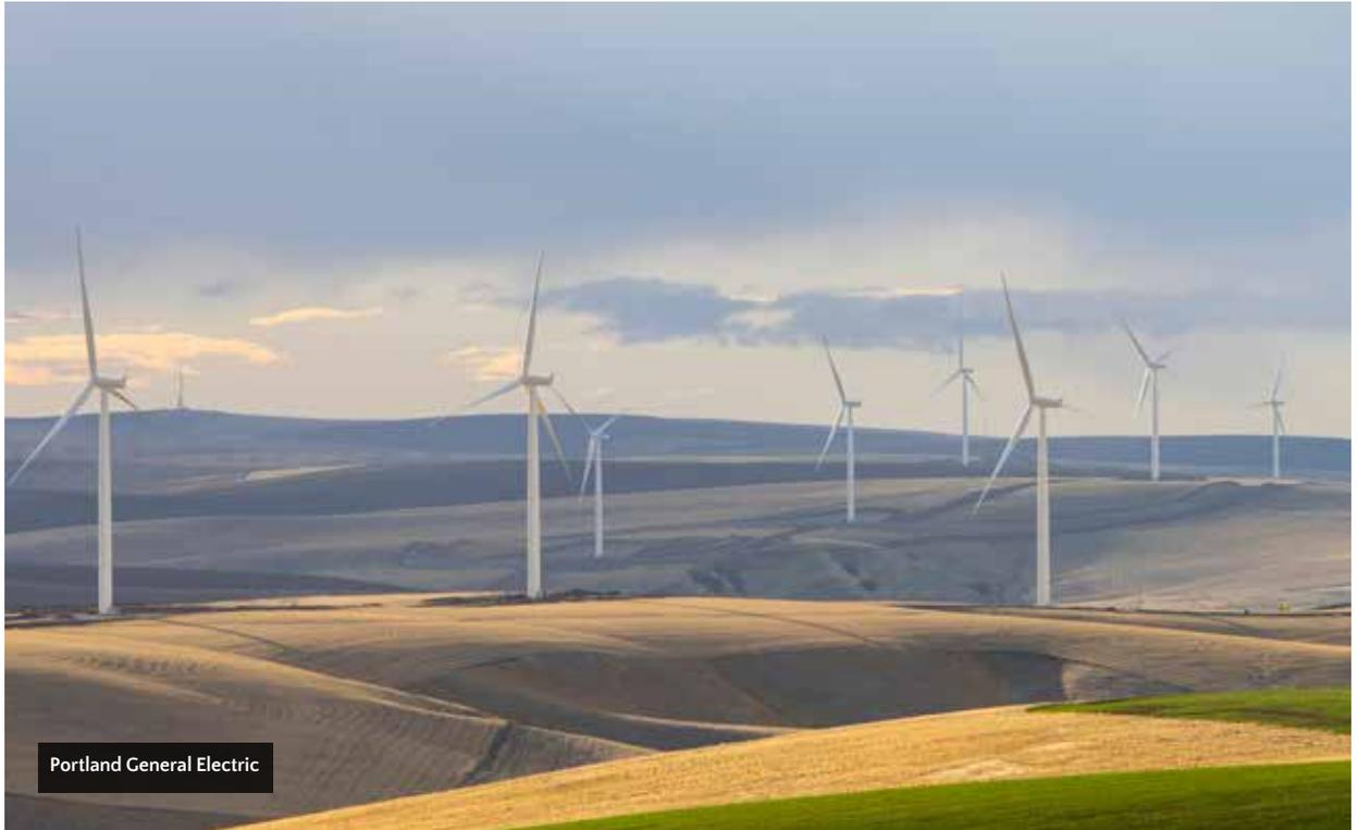
Portland General Electric Company recently announced its Tucannon River Wind Farm is in service and available to generate power for PGE customers. Tucannon River is PGE's second fully owned and operated large-scale wind project, with 116 turbines and a total installed capacity of 267 megawatts. Given the variability of wind power, the plant is expected to produce an average of 101 megawatts — enough to power the homes of about 84,000 average PGE residential customers.
