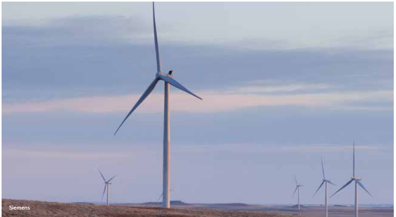
The Siemens SWT-3.2-101 and other models of the Siemens D3 product platform provide high energy yields and efficient operation for three Scottish onshore wind projects.
