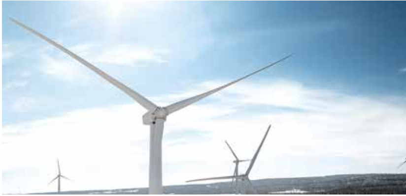
The battle against ice on blades will continue as wind-energy markets expand into colder regions. (Courtesy: LM Wind Power)
