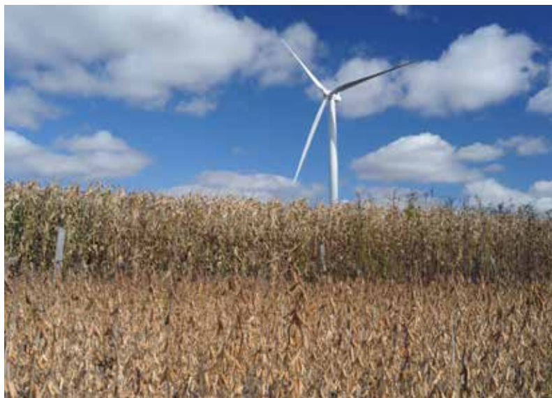
The Meadow Lake wind farm. (Courtesy: EDP Renewables)
