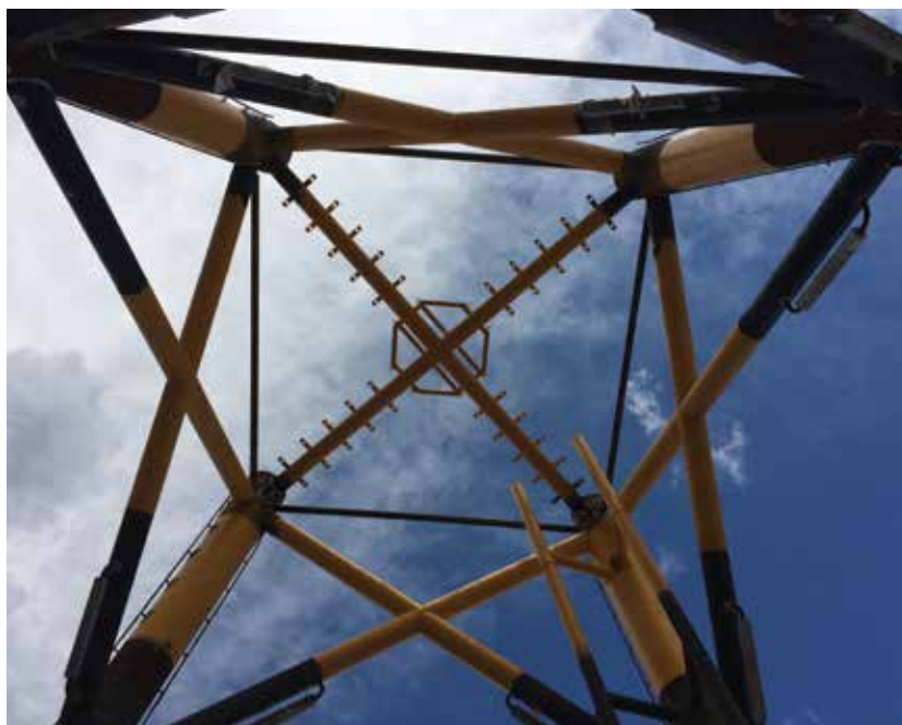
Gulf Island Fabricators constructed offshore wind turbine jackets for Deepwater Wind’s Block Island Wind Project off Rhode Island. (Courtesy: BOEM/Sid Falk)
