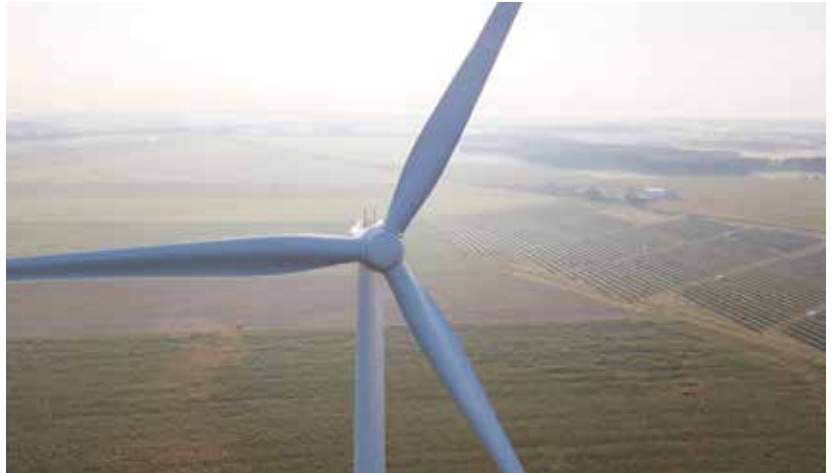
The SWT-DD-130 turbine features a rated capacity of 4.2 MW and a 130-meter diameter rotor. (Courtesy: Siemens Gamesa)
