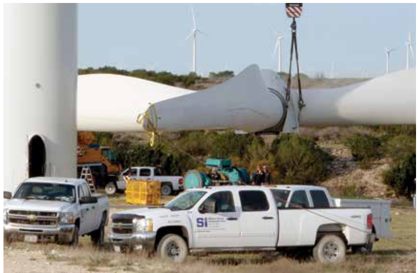
Field service generator replacement. (Photos courtesy: Shermco Industries)
