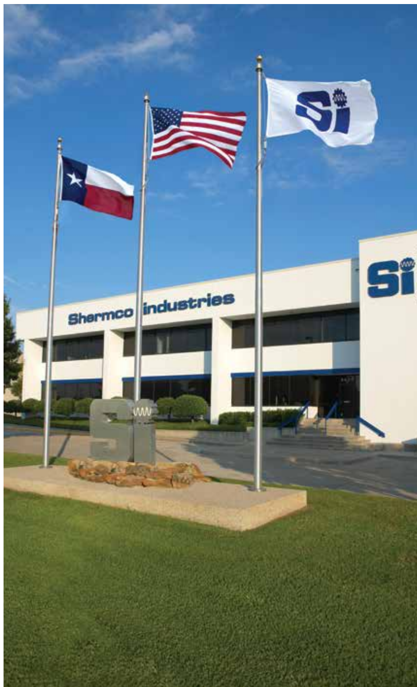
Shermco Industries’ corporate office and flagship remanufacturing center in Irving, Texas.
