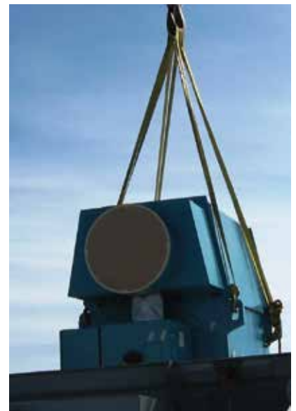
Generator being installed in turbine.
