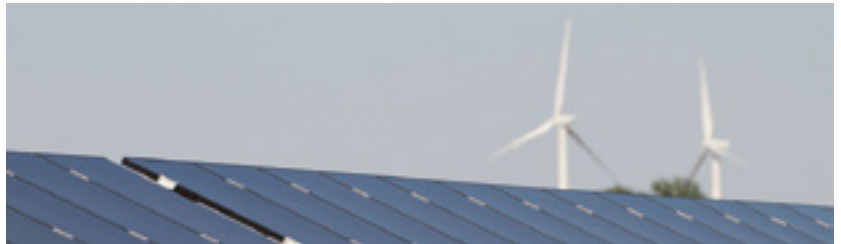
A 4.6-MW community-based project in Red Lake Falls, Minnesota, developed by Juhl Energy, uses two 2.3-116 wind turbines from GE Renewable Energy's Onshore Wind business supported by 1MW of solar power conversion equipment provided by GE's Current business. (Courtesy: GE Renewable Energy)
