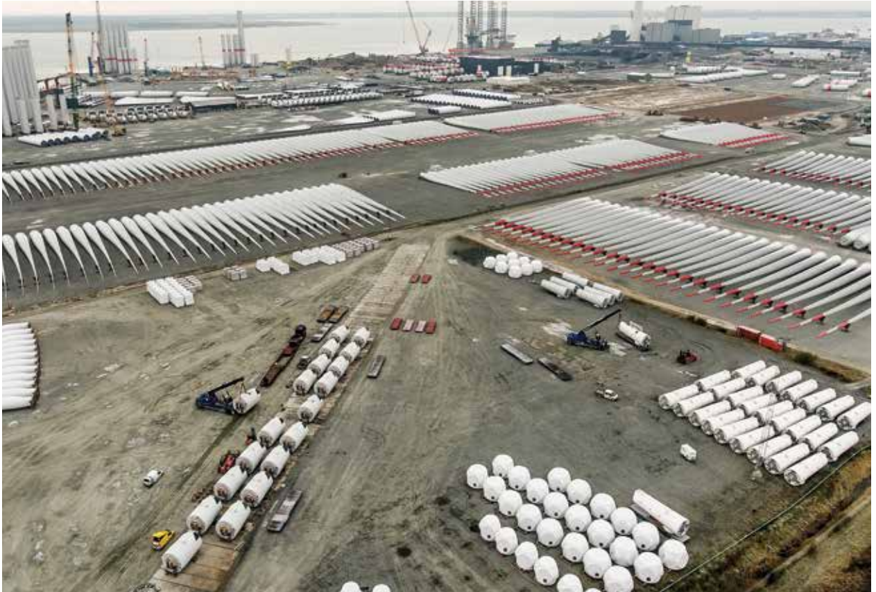
The Port of Esbjerg in Denmark is one of several offshore wind port “hubs.” (Courtesy: Port of Esbjerg)
