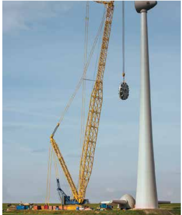
The Demag CC8800-1 can be used for wind-turbine installations. (Courtesy: Terex)
