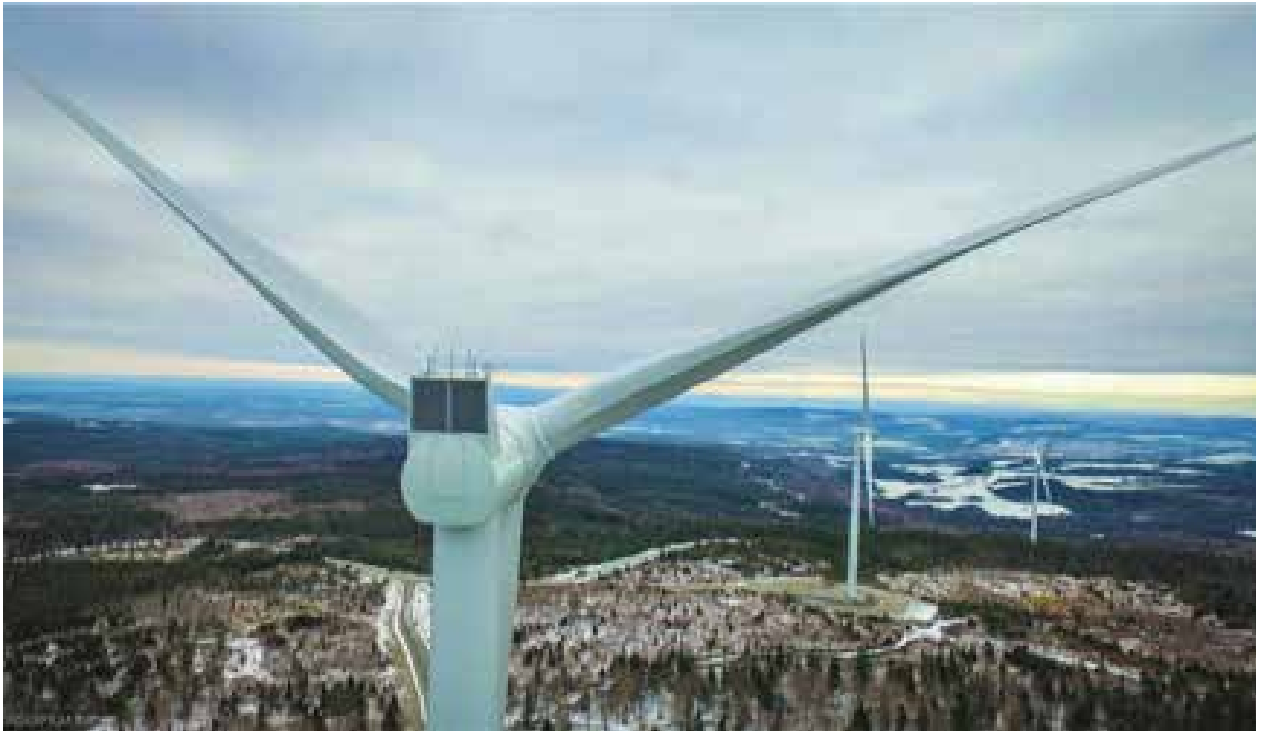
Turbine top view at Mont Sainte-Marguerite Wind. (Courtesy: Pattern Development)
