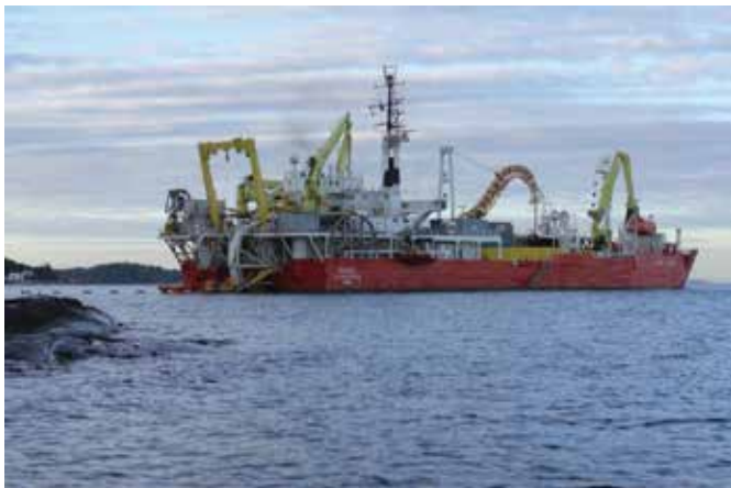
The Nexans-operated Skagerrak is responsible for laying the subsea export cables. (Courtesy: Beatrice Offshore Windfarm)
