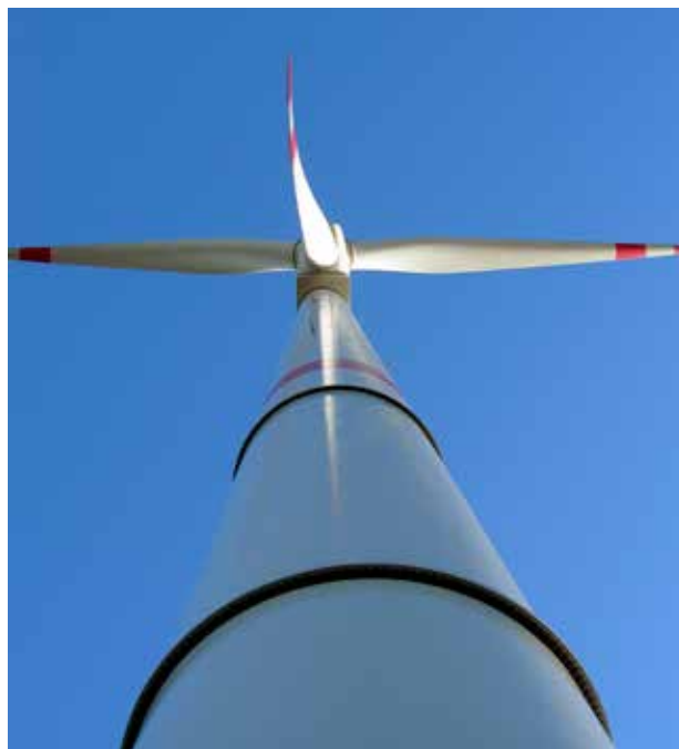
When mounted in key positions on mechanical equipment, vibration sensors offer continuous monitoring and analysis. While this requires investment, it is minimal when compared with the potential cost of downtime on a wind turbine. (Courtesy: Hansford Sensors)
