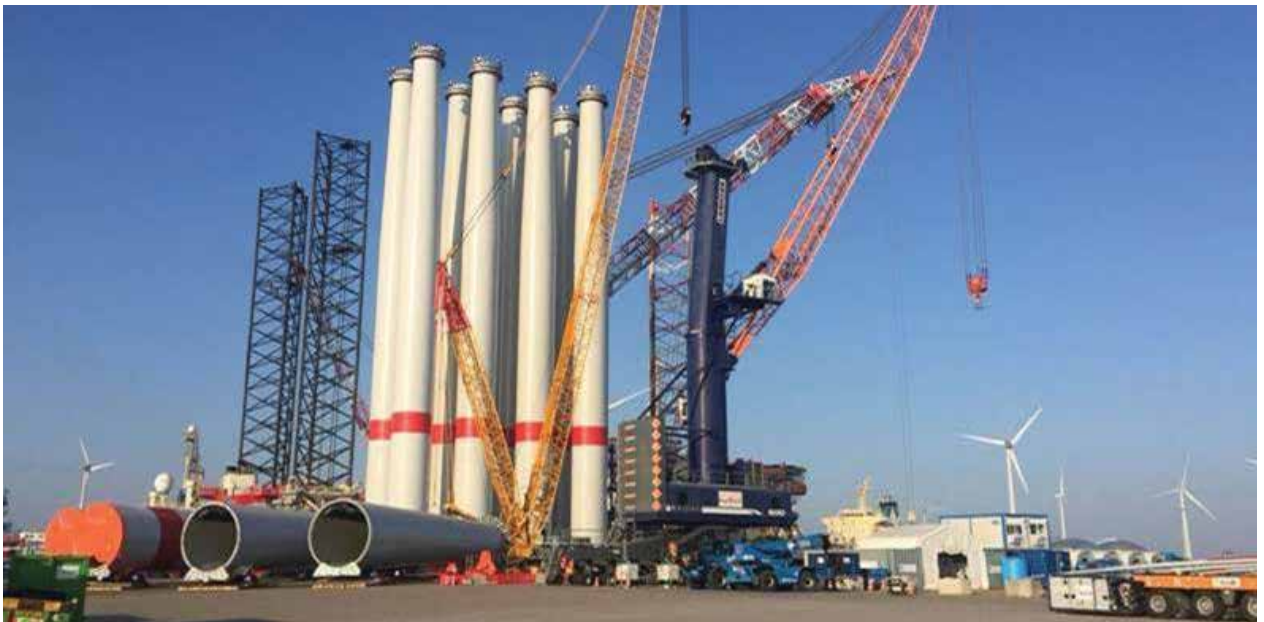
The pre-assembly of 66 Haliade 150-6MW turbines is part of the Merkur Offshore Wind Farm contract. (Courtesy: Gould Services)
