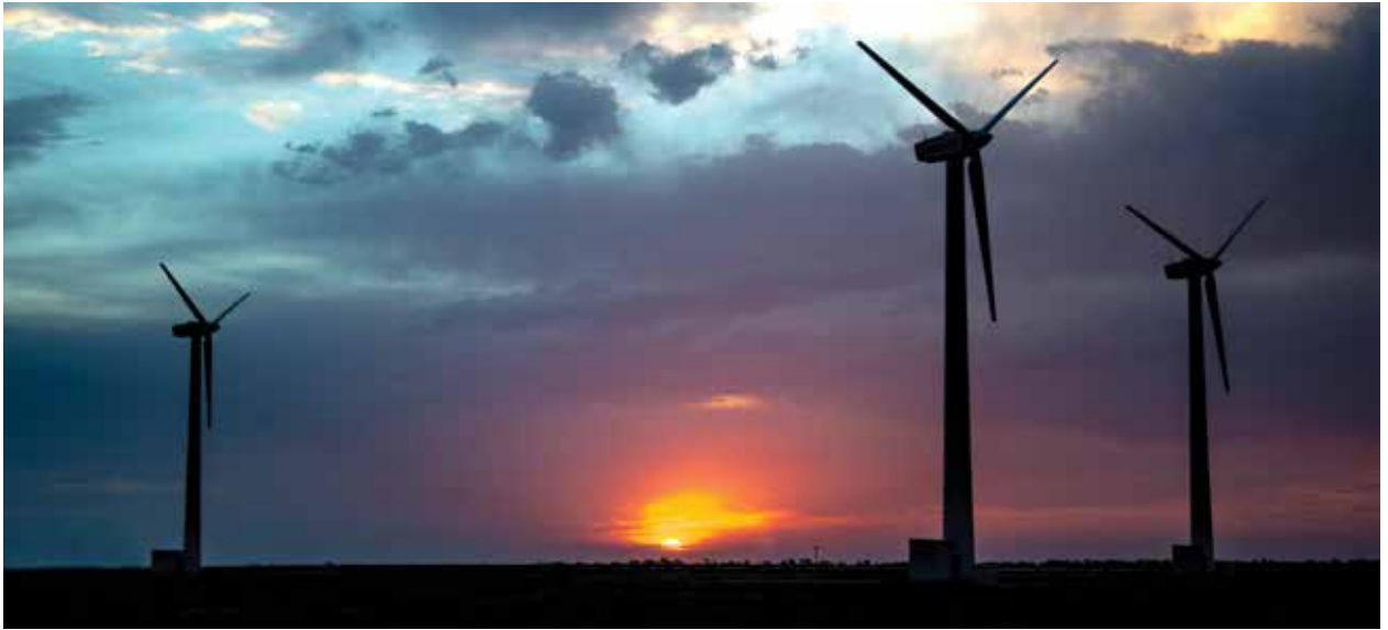
The SWiFT facility owned and operated by Sandia National Laboratories. (Courtesy: WindSTAR)
