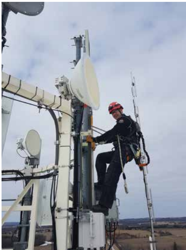
Inspecting a ladder fall protection system on top of a water tower.
