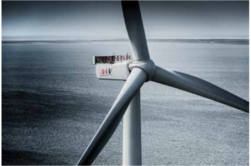
Moray Offshore Windfarm (East) Limited, known as Moray East, is a 950 MW offshore wind project 22 kilometers from the coast of Scotland. (Courtesy: MHI Vestas)
