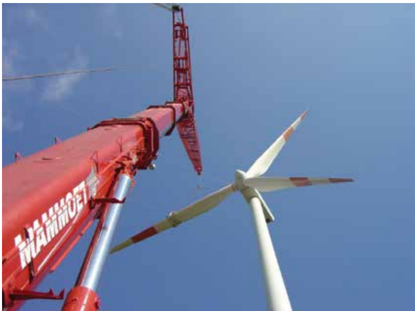
Mammoet helps clients improve construction efficiency and optimize uptime. (Courtesy: Mammoet)
