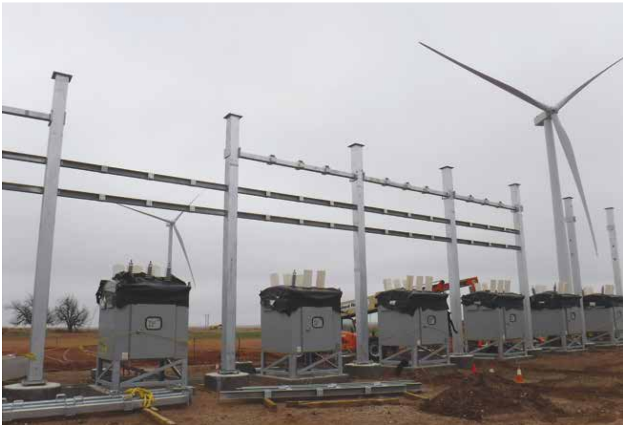
Wind farm substation construction. (Courtesy: Harvest Energy Services)
