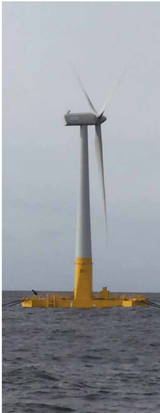
Floatgen is kept in place by a mooring design using clump weights designed and manufactured by FMGC. (Courtesy: Farinia Group)
