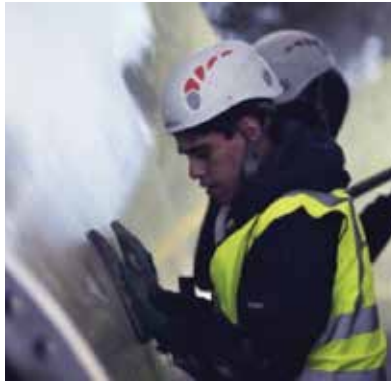
Three-quarters of Altitec’s inspections and repairs around the world were carried out on wind farms younger than 5 years old. (Courtesy: Altitec)
