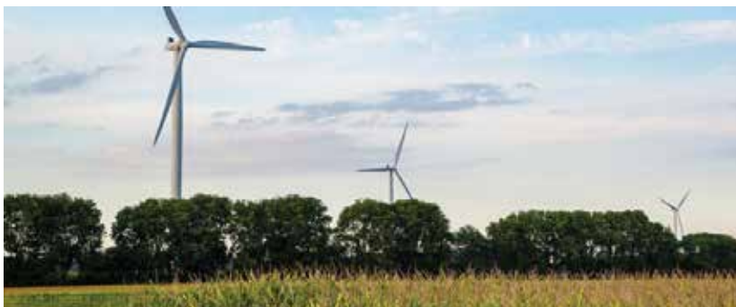
Sugar Creek Wind is an advanced-stage 202 MW project. (Courtesy: Apex Clean Energy)
