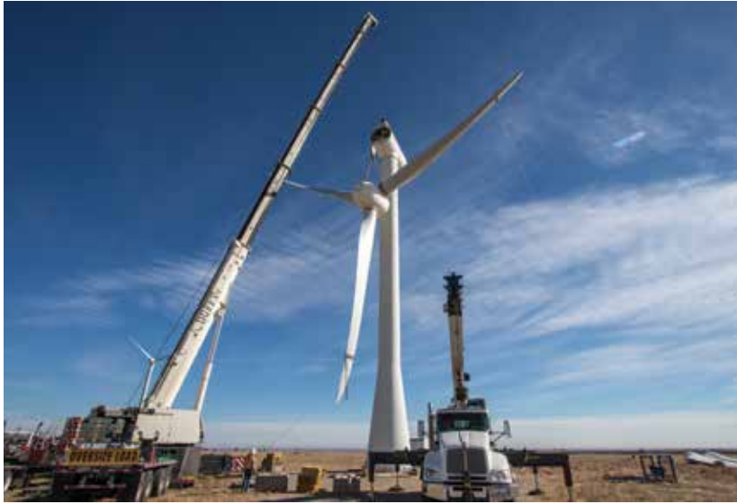
Installation of the “SmartBlades2” rotor blades. (Courtesy: Lee Jay Fingersh, NREL)
