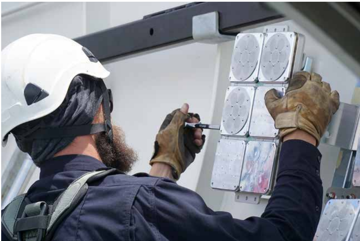
A Bat Deterrent System being installed in Hawaii for testing.
