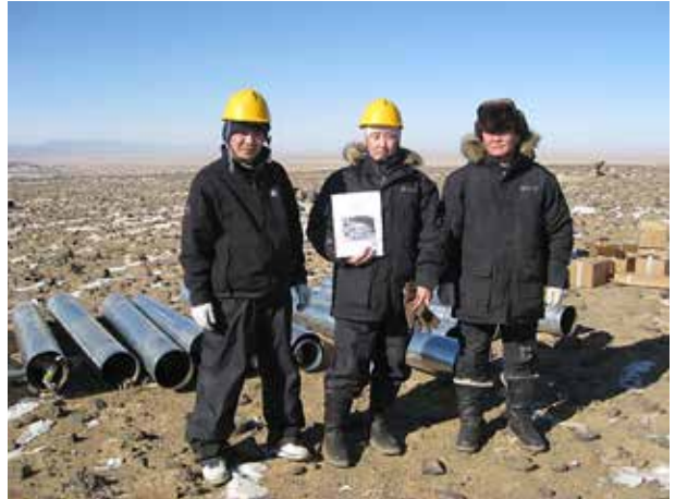
NRG tower installation in Mongolia.
