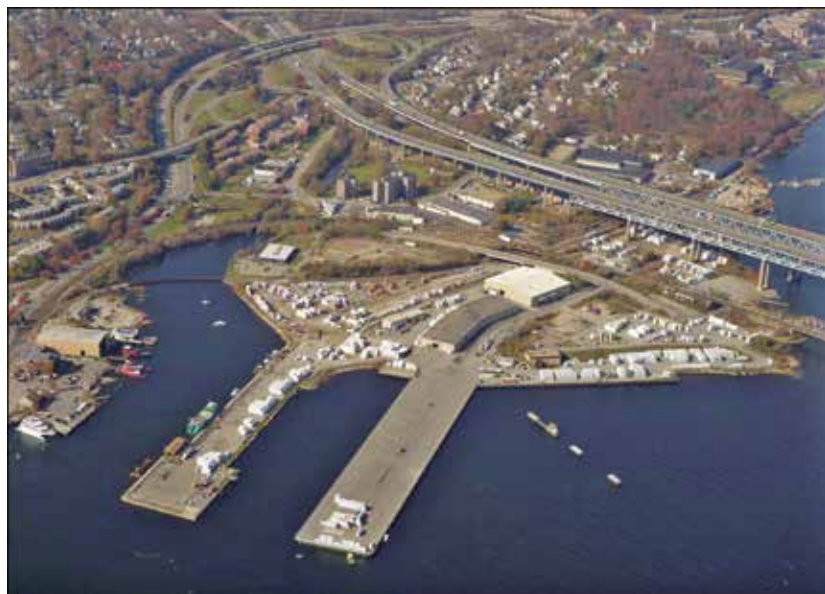
State Pier in New London Connecticut. (Courtesy: State of Connecticut)
