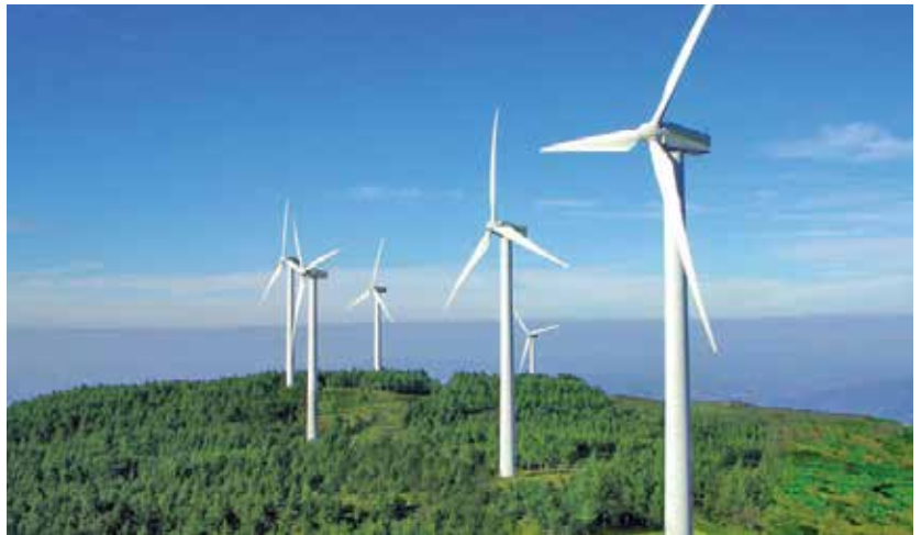
Some wind farms are using the data collected from their systems to predict when faults will occur and schedule maintenance before it’s needed. (Courtesy: Clobotics)
