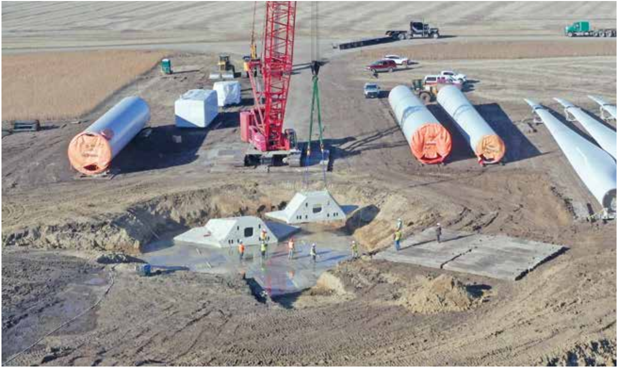
The RUTE system is stronger than standard concrete, so wind farms can upgrade to larger towers without additional costs. (Courtesy: RUTE Foundations)
