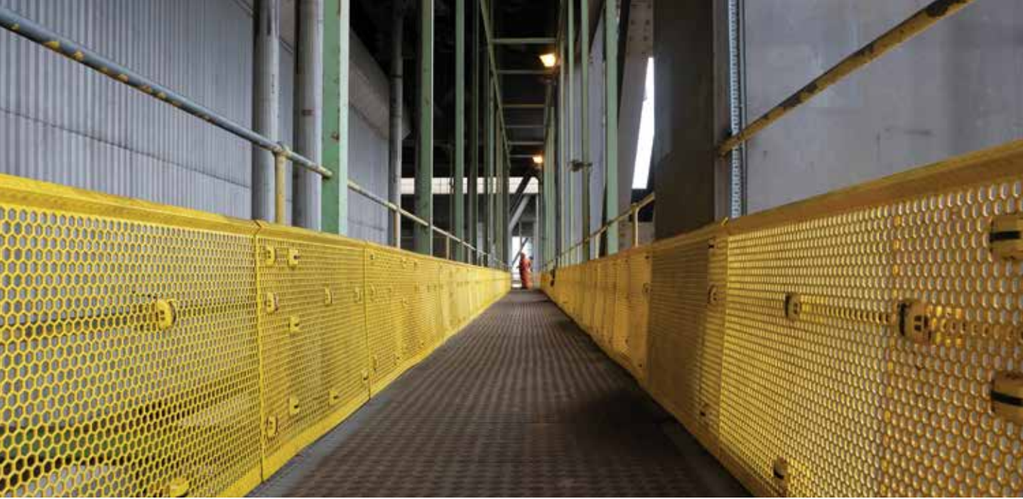
The Dropsafe Barrier installed at a power generation facility in Asia. (Courtesy: Dropsafe)
