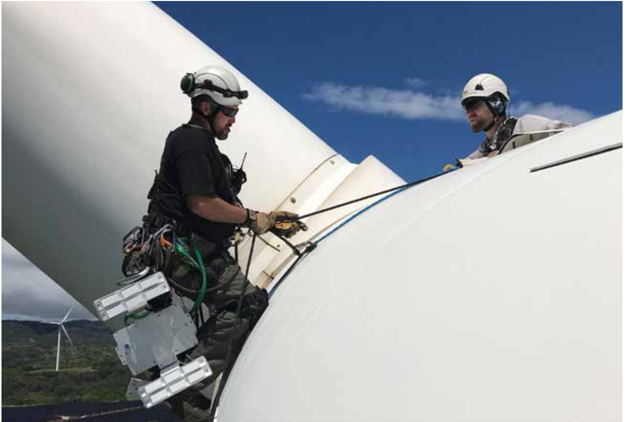
Kawailoa Wind is installing NRG Systems' Bat Deterrent System on its 30 turbines. (Courtesy: NRG Systems)
