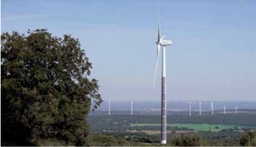
The system has been installed in one of the turbines of the Breña Wind Farm in Albacete, Spain. (Courtesy: Acciona)
