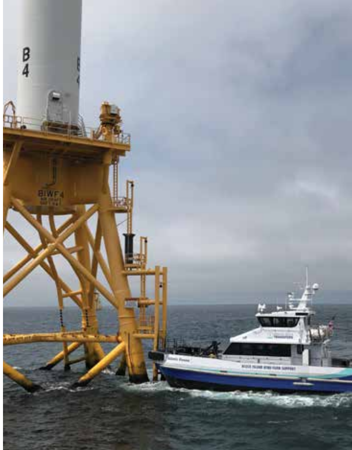
A 6-MW offshore wind turbine like the ones at Block Island can power approximately 2,300 homes, and manufacturers are working on even more powerful models above 10 MW.
