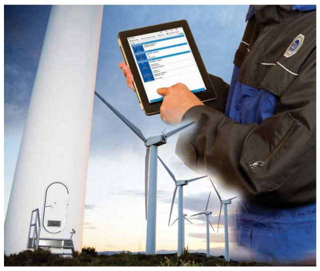
The lifetime extension assessment thus consists of two parts: an analytical evaluation and an on-site inspection. (Courtesy: TÜV SÜD)
