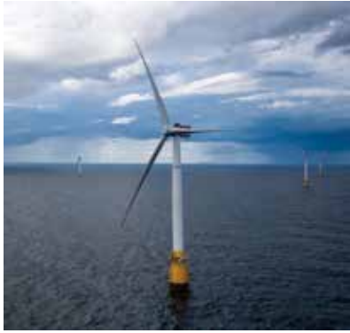
In Norway, Equinor will implement design and installation learnings gained since its Hywind Scotland project came online in 2017. (Courtesy: New Energy Update)
