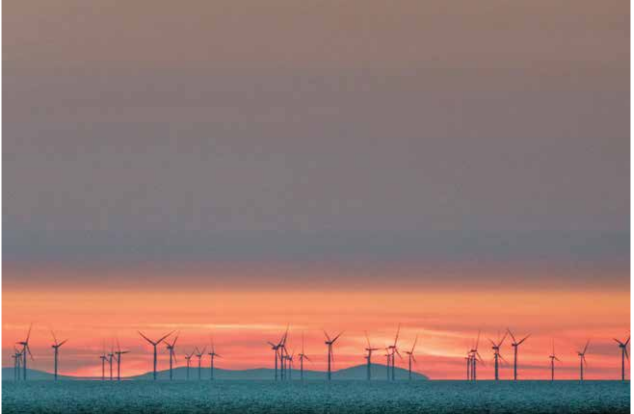
Siemens Gamesa offshore project. (Courtesy: Siemens Gamesa)
