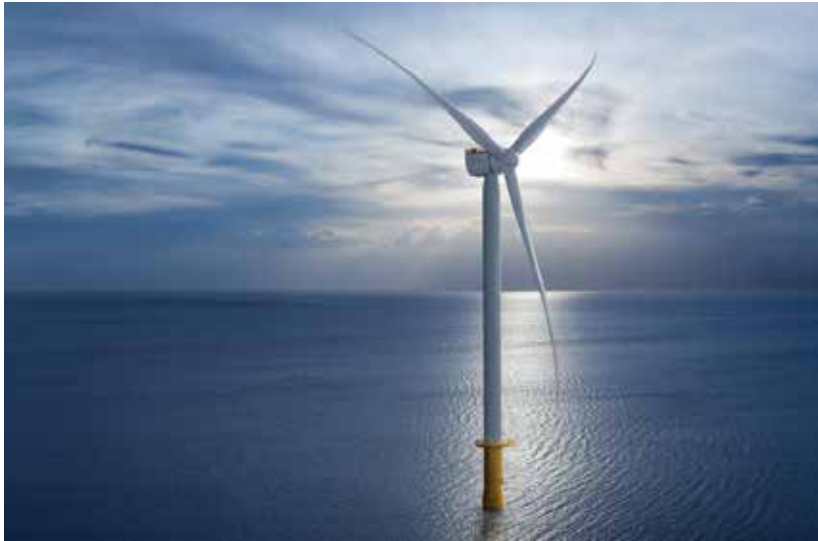
The SG 11.0-193 DD Flex offshore wind turbine features a 193-meter diameter rotor using the 94-meter long Siemens Gamesa B94 Integral Blades. (Courtesy: Siemens Gamesa)
