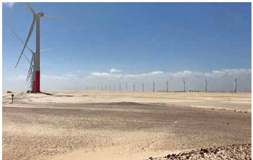
Due to an extremely corrosive environment, a wind farm in Brazil was having significant corrosion issues which were successfully overcome by applying VpCI® Technology. (Courtesy: Cortec)
