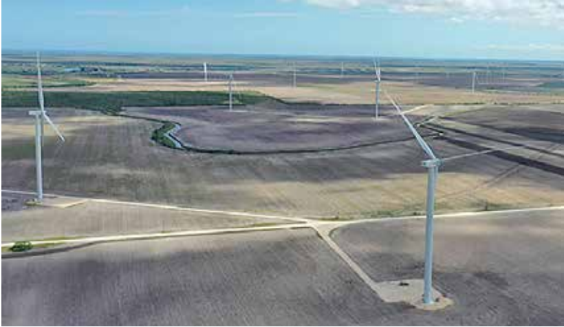
Palmas Altas wind farm features 46 Nordex technology wind turbines totaling 145 MW capacity. (Courtesy: Acciona)
