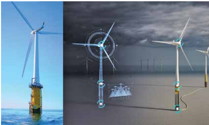
4Subsea has developed a new generation of sensors for structural integrity and performance monitoring of offshore wind turbines. (Courtesy: 4Subsea)
