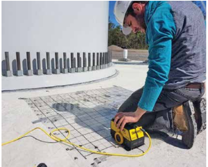
Figure 2: Ground-penetrating radar for rebar scanning.
