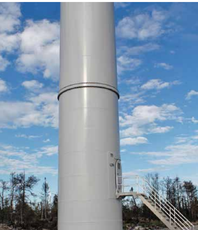
Figure 1: Concrete foundation of a wind-turbine structure.
