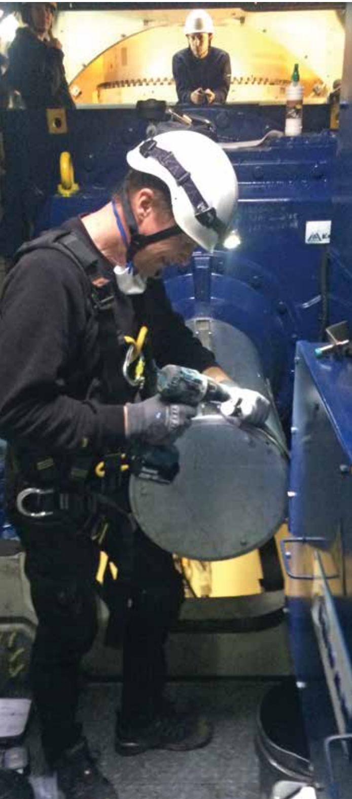
Inside a wind turbine nacelle during a “typical” site survey. (Courtesy: B&K Vibro)
