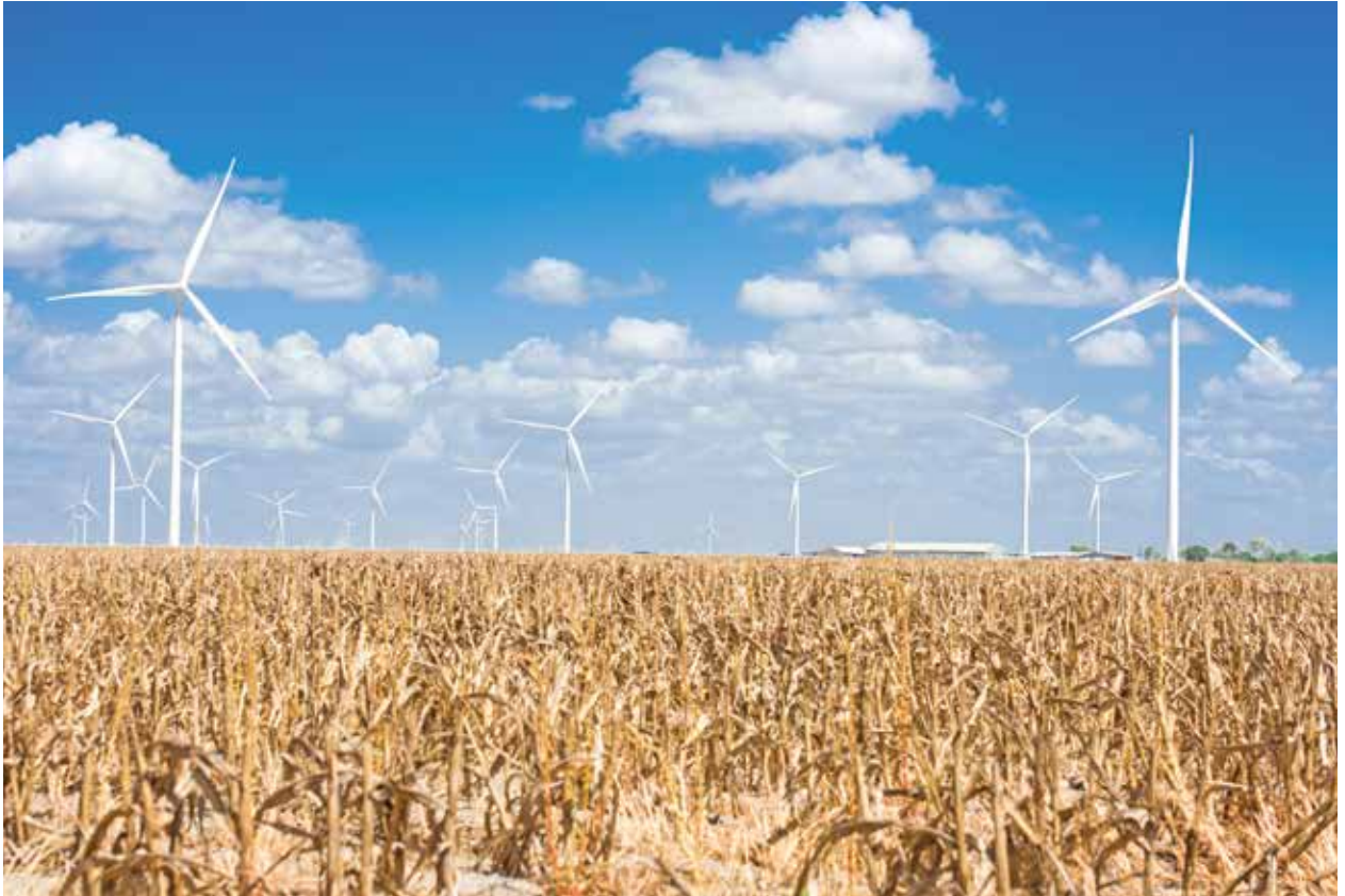
The Haystack project includes the supply of 51 SG 5.0-145 wind turbines and 18 safe harbor turbines. (Courtesy: Siemens Gamesa)
