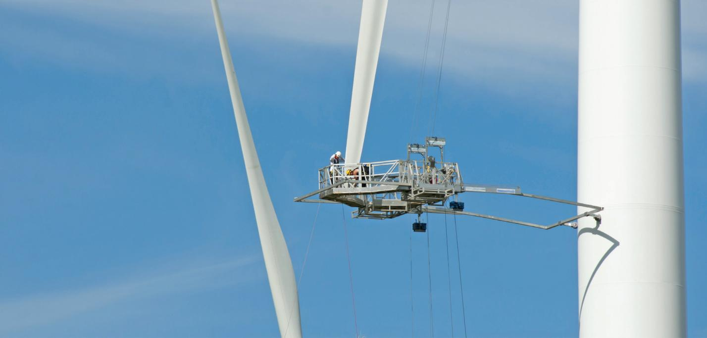
World Wind & Solar's newest services include gearbox exchanges, blade exchanges, and blade and composite repair. (Courtesy: World Wind & Solar)
