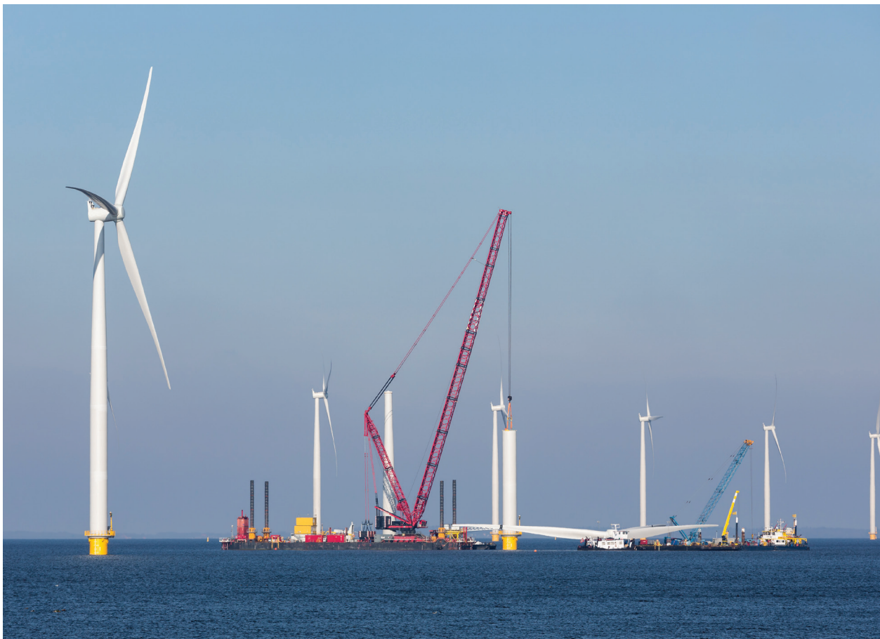
Fixed bottom WTG are installed in two stages: first the installation of the fixed bottom structure, then later, the deployment of the WTG using a jack-up installation vessel. (Courtesy: Shutterstock)
